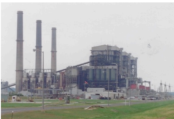
Electric Power Utility Plant Coal Fired Boilers
