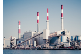
Electric Power Utility
